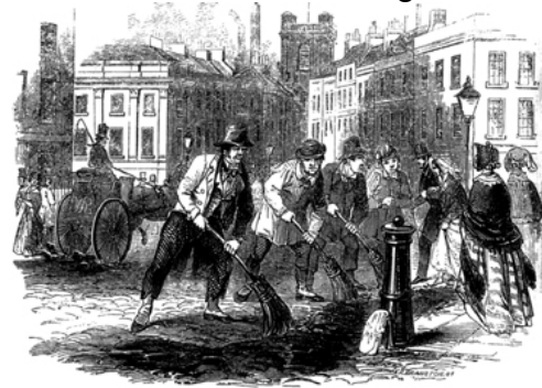
Workmen sweeping a newly-paved town street
